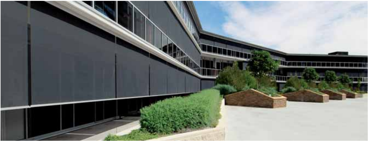
Solar activated blinds: the sun triggers sensors to lower the blinds—cutting heat-transfer and letting occupants open balcony doors to enjoy the resulting ambient air.
