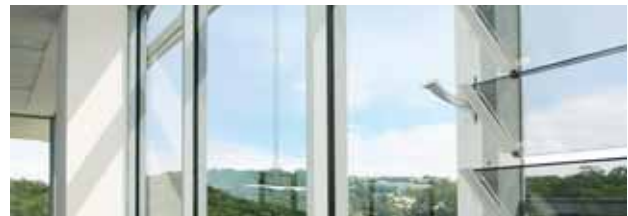
External louvres: fresh air and less need for air-conditioning.
