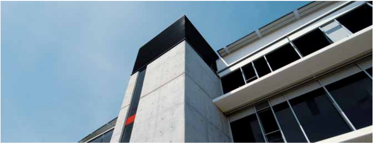
Stairwell and heat chimney: enables a natural flow of air through the building, reducing the need for air-conditioning.
